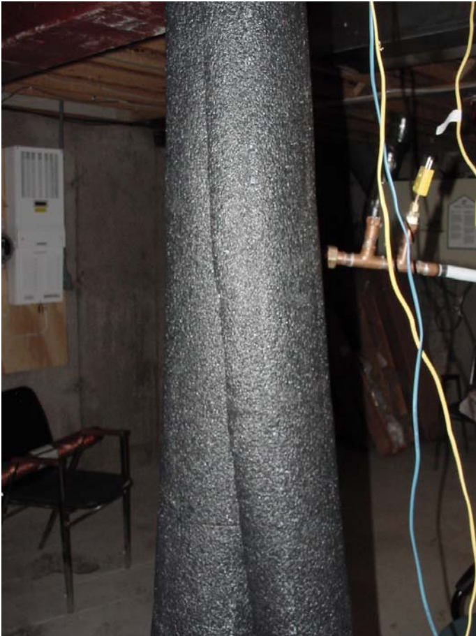
Figure 2: Insulated DWHR
