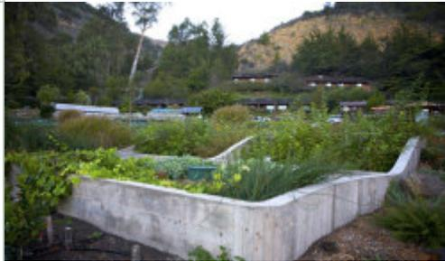
This "tidal-flow wetland" Living Machine treats wastewater from the laundry and lodging facilities at the Esalen Institute in Big Sur, California, for use in irrigation and aquifer recharge.
